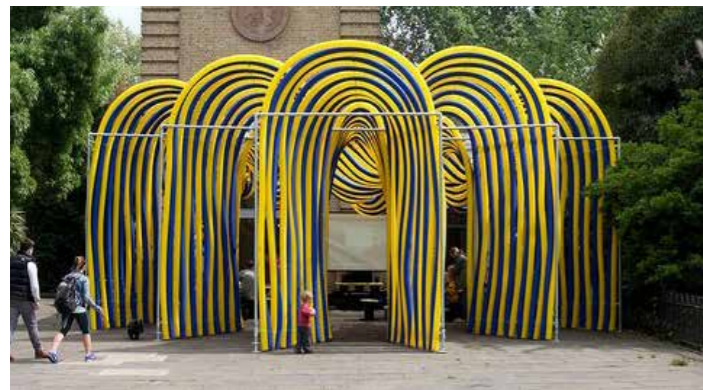
Pump House; part of the Wandsworth Fringe Festival
