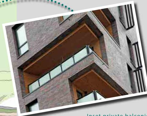
Brick detailing to mark the location of different flat types
