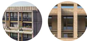
The top two floors reference the Alton Estate and are set back to provide shading to the apartments.
